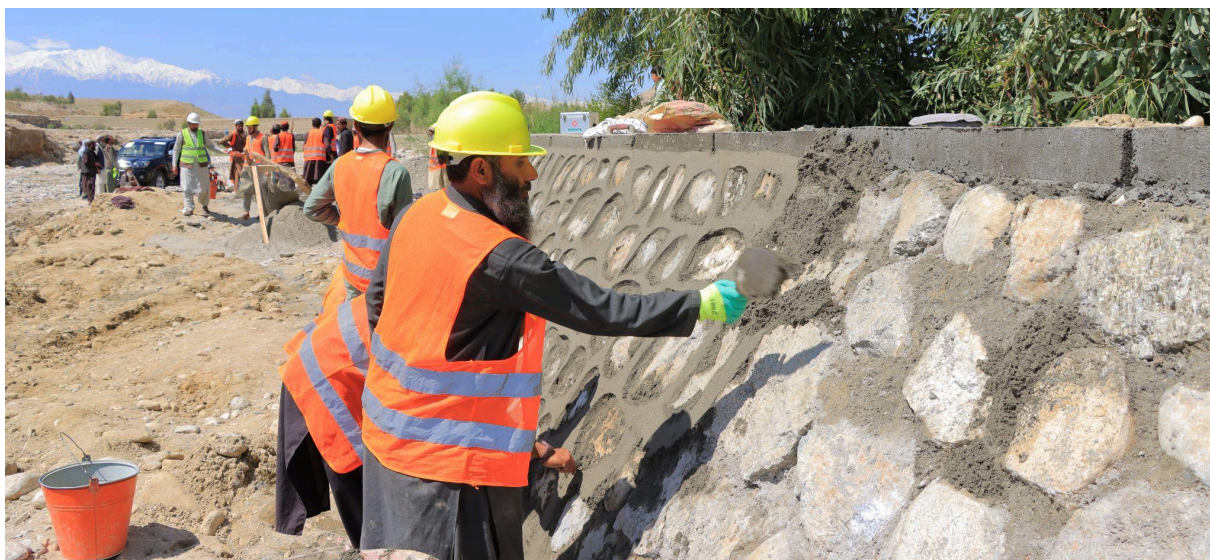
Photo: Construction of a 51 meter- long retaining wall in Kot District of Nangarhar Province on 6 May 2024.
