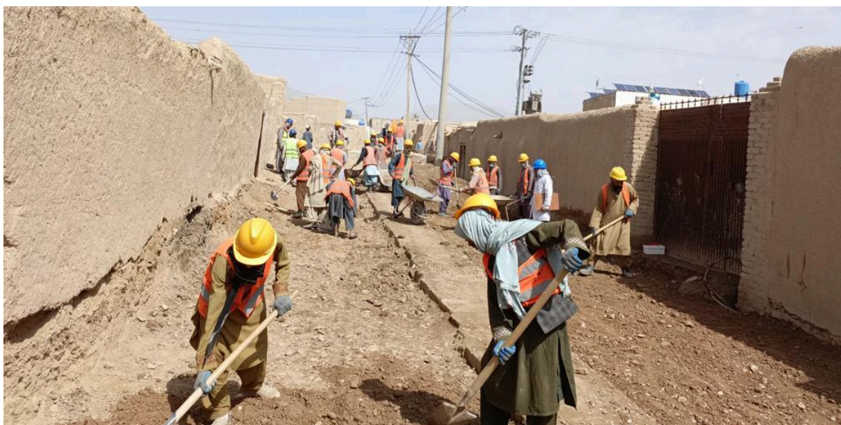
Photo: Construction of Plum Concrete Surface Street in District 12 of Kandahar Province on 23 May 2024 by laborers
